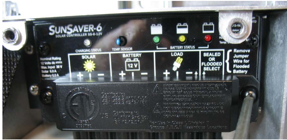
Figure 5-9: Removing the Termination Cover (if present)
