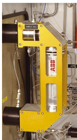
Extractive Analyser Sample System for Final Product Blending Application
