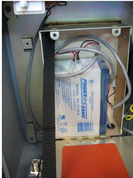
Figure 2-30: Battery Pack Attached to Compartment
