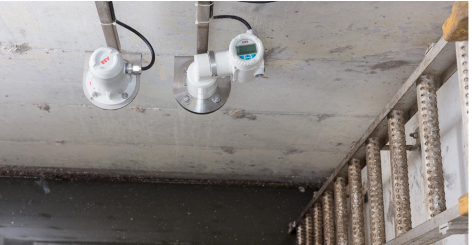
01 ABB laser level transmitters used in municipal wells to measure wastewater level.
