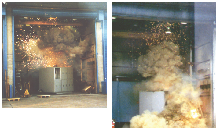
Conventional switchgear 50 kA interruption at KEMA Test Lab
