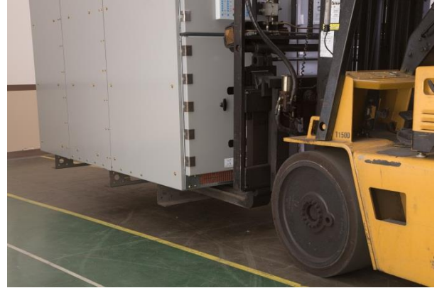
Figure 5: Lifting of switchgear frames with forklift
