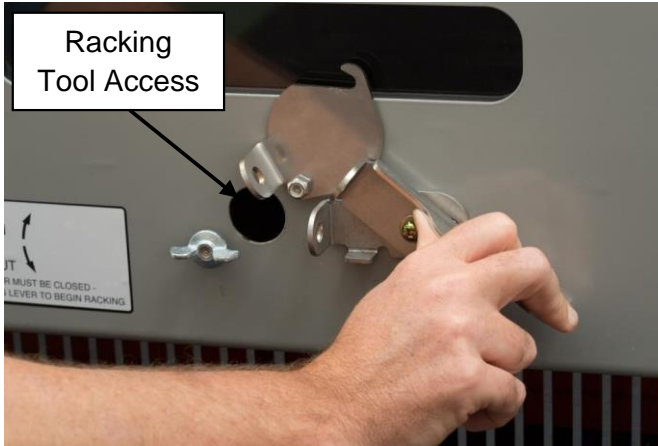
Figure 21: Racking release handle
