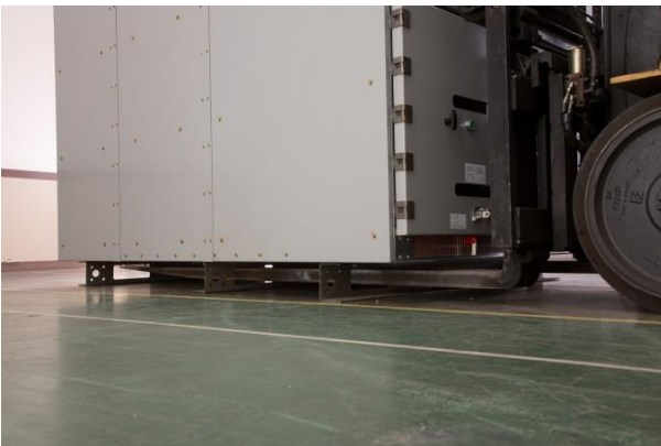
Figure 4: Complete fork penetration of all 3 shipping channels
